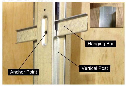
The Vertical Posts are cut on site. If a site condition requires the post to be cut down in length ALWAYS cut from the bottom.
